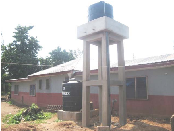
Photo – left: the water tower and tank for the electric borehole in front of the four new rooms built for the Offia Oji health center. Photo – right: some of the staff in front of the new staff quarters at Offia Oji.
